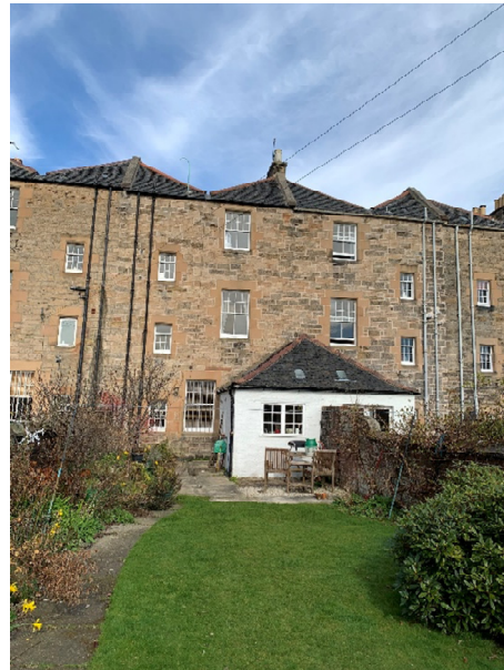
Rear Elevation of 18 Inverleith Gardens
